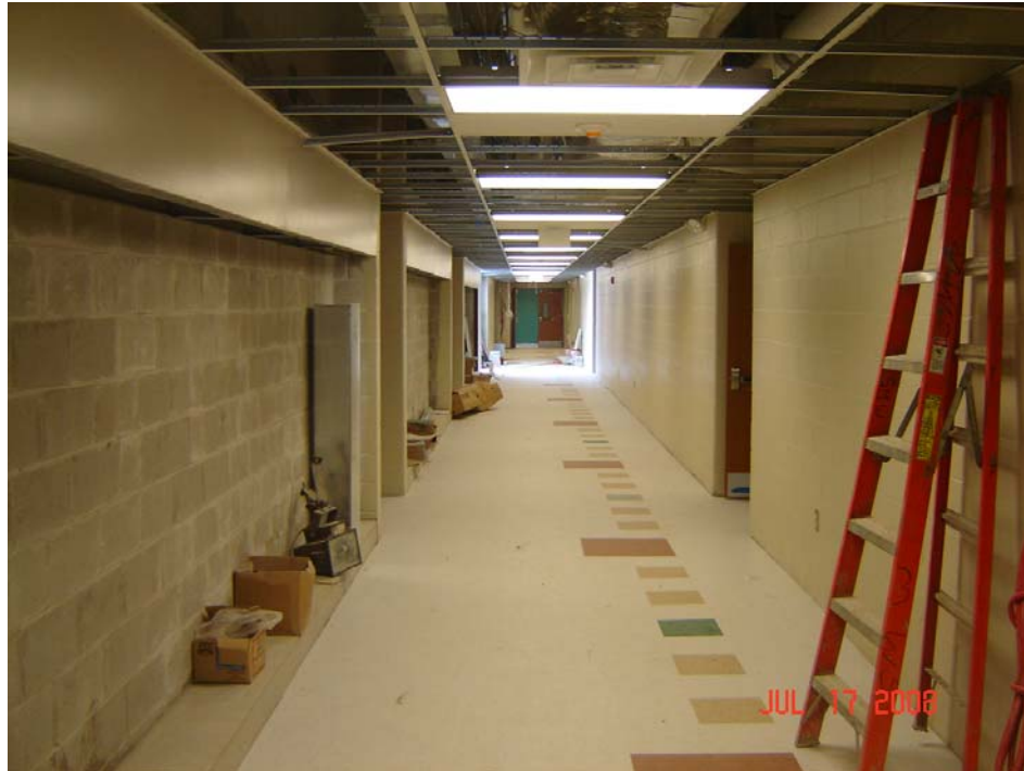
Third floor corridor.
