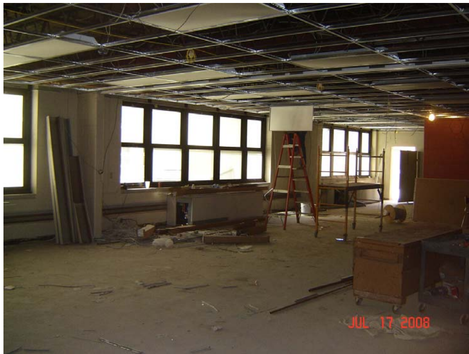
Renovation work at Cafeteria Anex.
