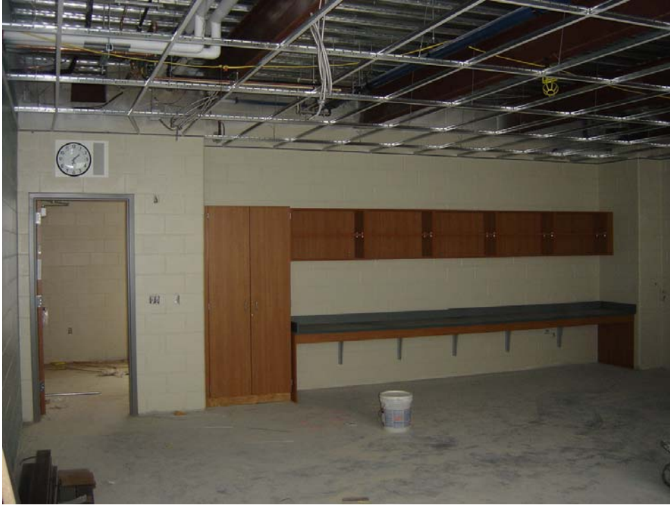
Installation of finishes at a typical classroom.
