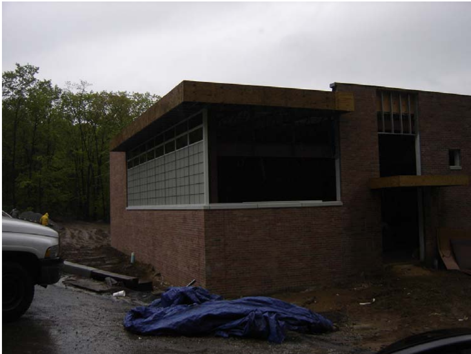
Window installation at Music Room.
